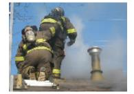
released from the interior of the structure, allowing firefighters to reach the seat of the fire and quickly extinguish the fire. Whenever a hole is necessary, we always cover the hole using roofing paper and tacks in an attempt to prevent water leakage.
